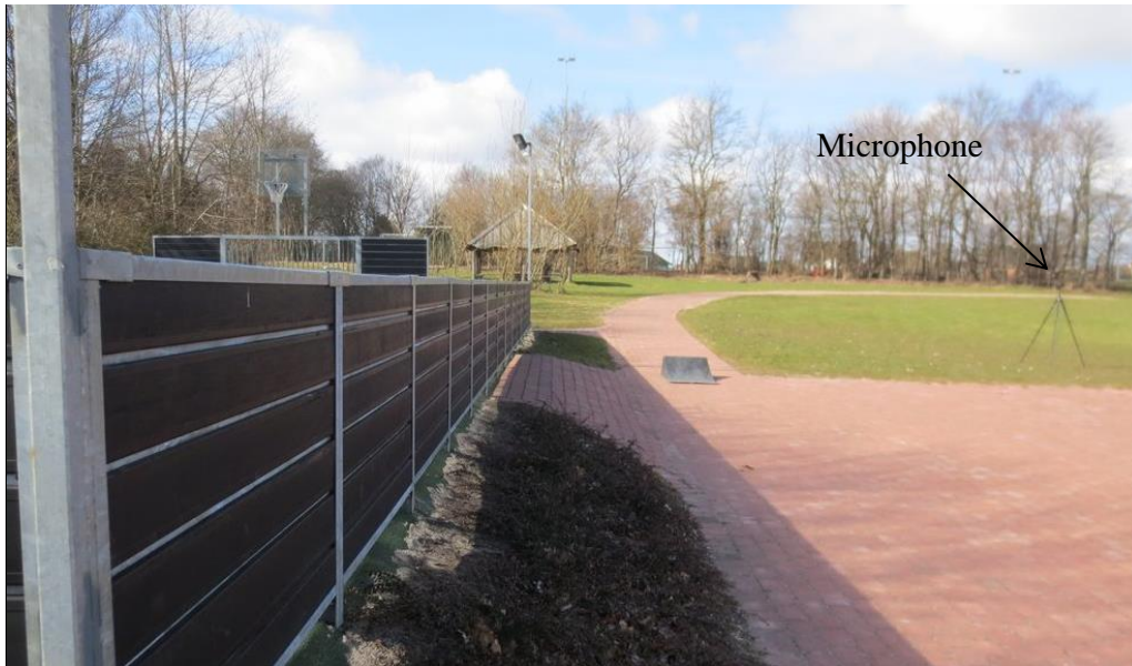
Figure 3 Photo of the fence and the microphone (shown from east).
